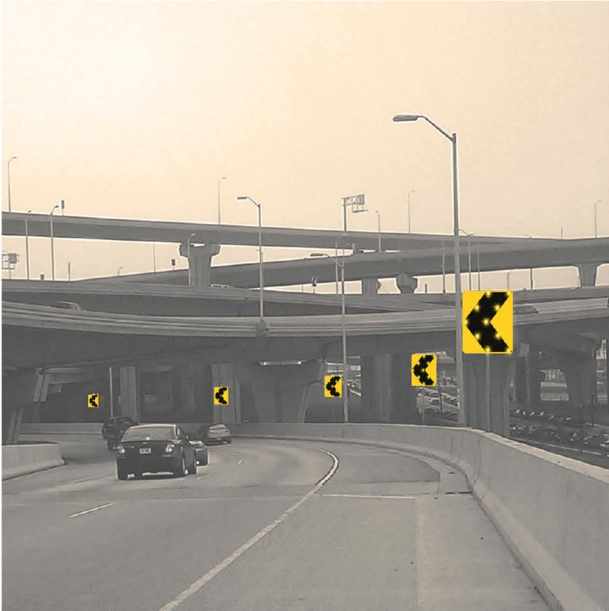
BLINKERCHEVRON™ DYNAMIC CURVE WARNING SYSTEM
